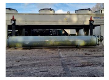
HELPMAN Groningen Holland Pressure vessel type 13-15-335-4KIP Shell side | Tube side Test pressure 25 bar bar 5 23 bar king 3 22
